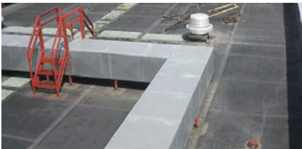
□ Before - EPDM roof
