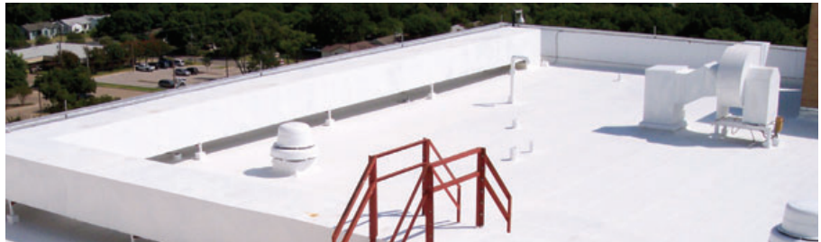
□ After - StressPly SA coated with Pyramic
