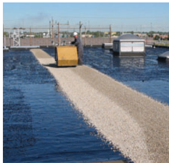
□ Gravel being applied over WeatherScreen
