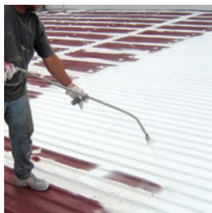
Protecting your metal roof with Rust-Go and White-Knight/ White-Stallion spray application
