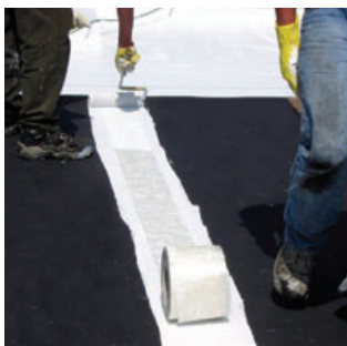
Single-Ply with White-Knight/ White-Stallion reinforcing the seams
