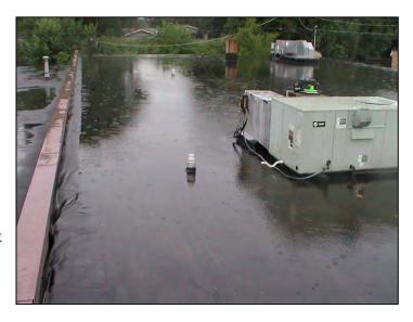
In most cases, secondary drainage units must have a separate outlet in addition to the primary unit. This outlet should be above grade and in a location that can be seen by building occupants. It should also be noted that if scuppers are used for the secondary drain system, they should be sized and located to prevent ponding water from overloading the structure if the primary system were to back up.
