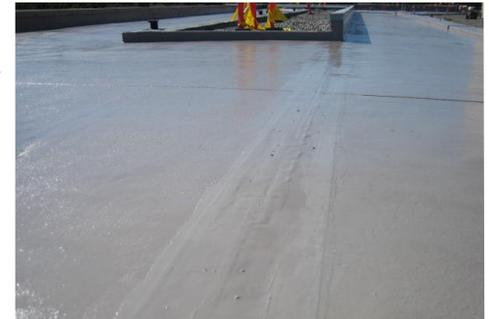
Hybrid Sealant installed in large parking deck expansion joint
