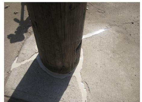
*Hybrid Sealant installed in prepped Concrete Surface with cracks and spall damage due to ice and UV degradation*
