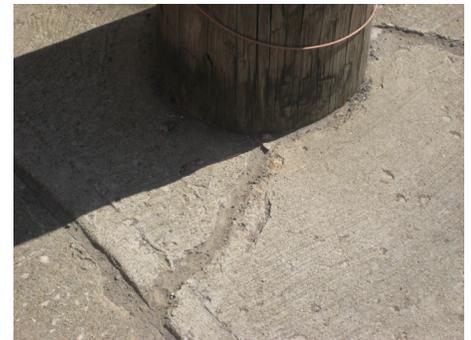
*Prepped Concrete Surface with crack and spall damage due to ice and UV degradation*
