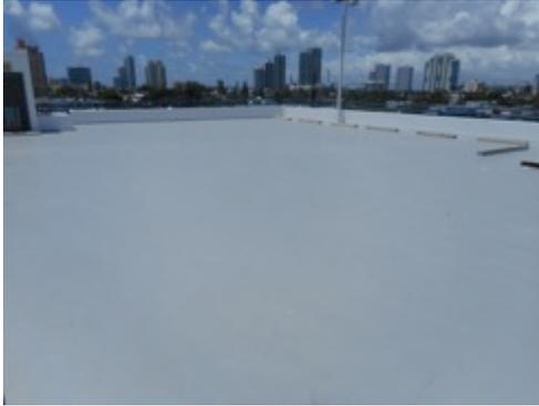
The city has a diligent preventive maintenance program that requires buildings to be inspected yearly. As a part of that maintenance program, a building envelope and structural analysis was conducted. It was determined that the parking garage's horizontal and perimeter joints were failing, allowing water to enter the building. Additionally, the waterproofing for the vehicle impound area had completely worn away or failed in many areas.
