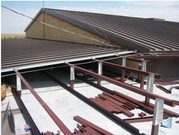
Typical Retrofit Metal Roof & Framing System
