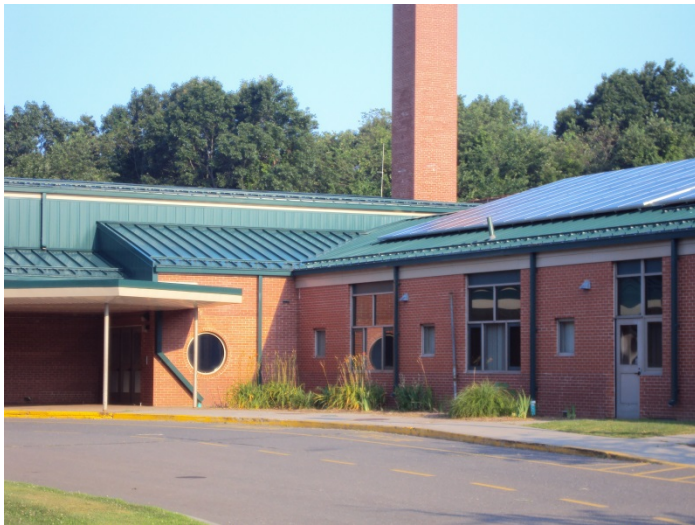
Solar Installation over a Retrofit Metal Roof
