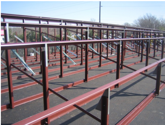
Temporary Roof under a Framing System
