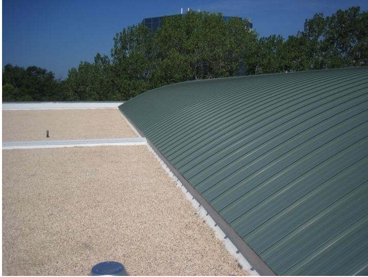
New Retrofit Metal Roof with Replacement Low Slope Roof Area
