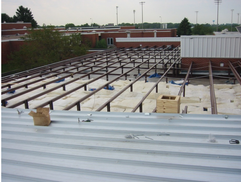
Retrofit Metal Roof with Insulation
