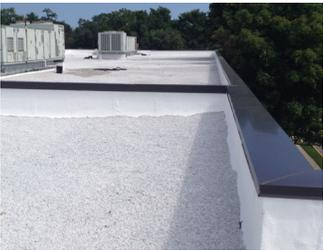
The new system was installed using Garland's Weatherking® cold-process, VOC-compliant adhesive with StressPly® EUV eco-friendly, fiberglass-polyester reinforced modified bitumen membrane installed as the cap sheet. The system was then coated with flood and gravel to provide additional waterproofing and UV protection. The flashings were coated with a highly reflective, ENERGY STAR® qualified acrylic coating, providing added UV protection, reduced heat gain and a clean, consistent surface.
